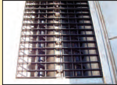
Dual Auger with Bottom Screens
